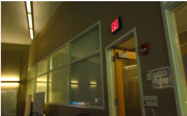
Interior Window that Staff Would like Removed
