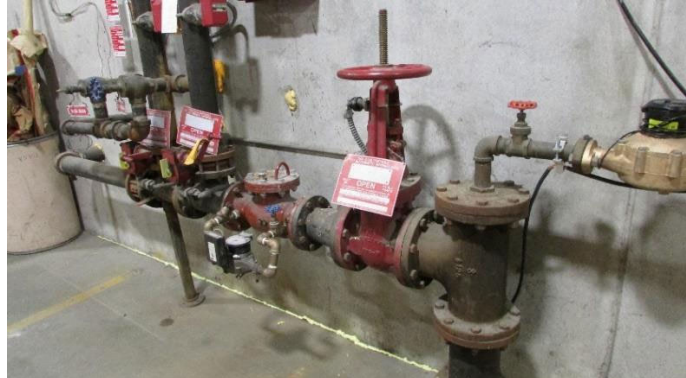
6" Water Sup Srvs Potable Water/Fire Sprinkler Systems
