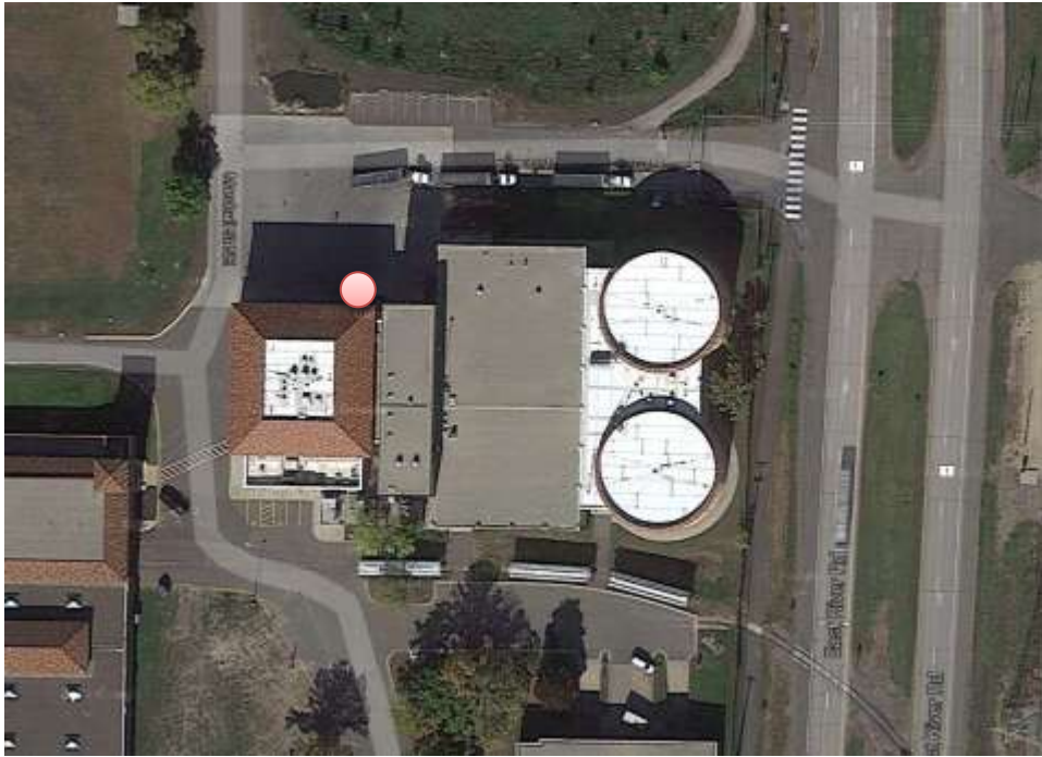
Fridley Dewatering Facility
