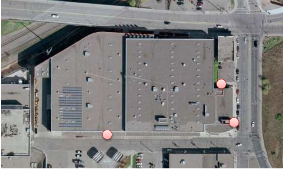
Currie Maintenance Facility
