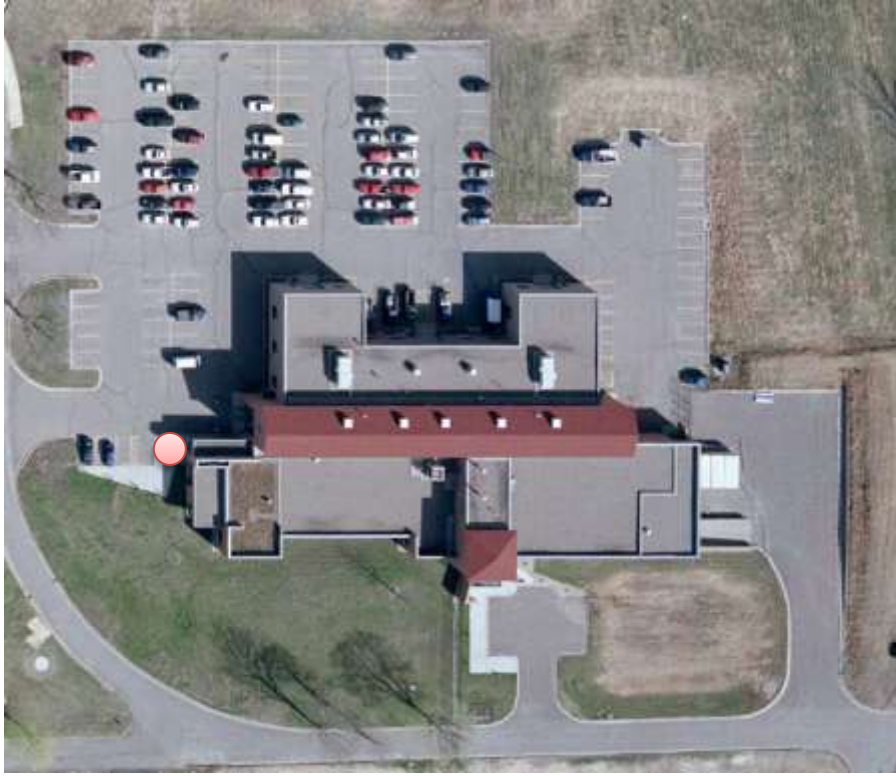
Fridley Maintenance Facility
