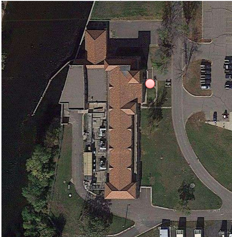
Fridley Pump Station 5
