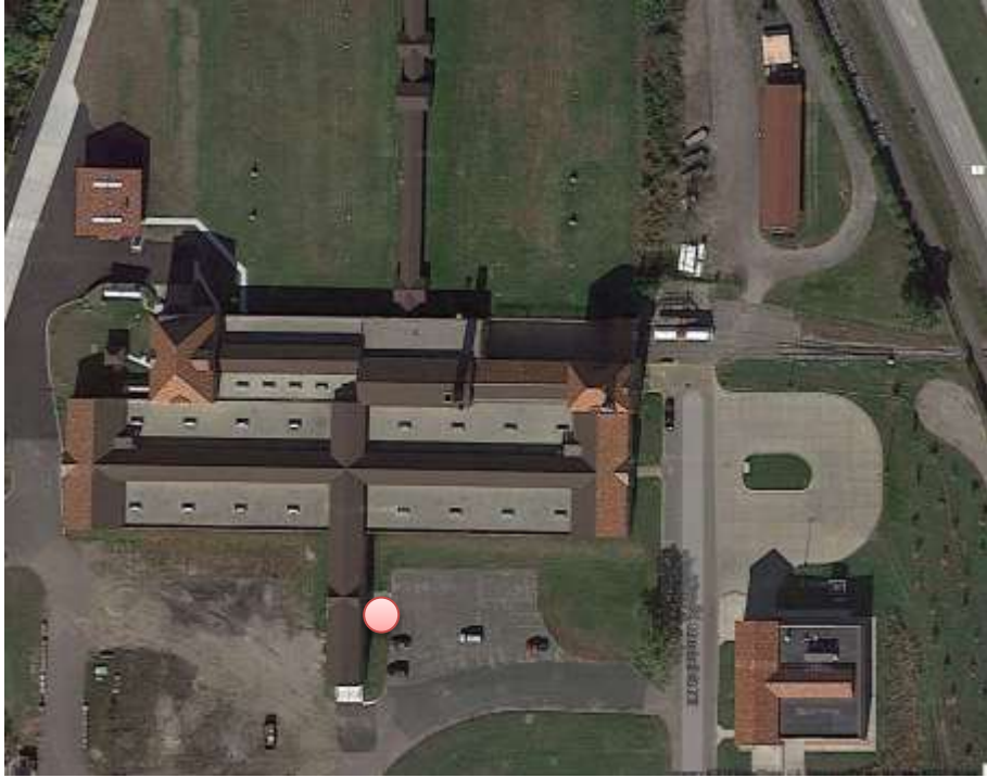
Fridley Filter Plant
