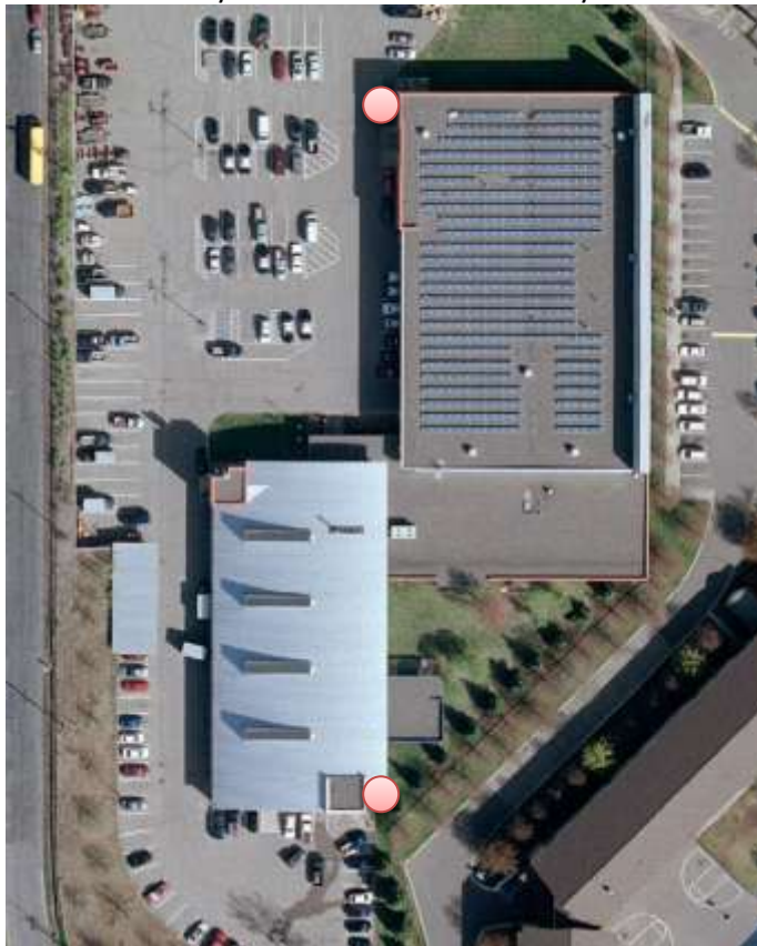
Royalston Maintenance Facility
