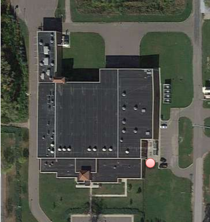
Columbia Heights Membrane Filtration Plant
