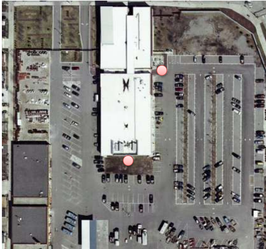
Hiawatha Maintenance Facility
