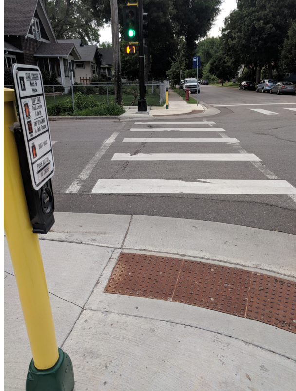
Figure 3-9: Push buttons and pedestrian signal heads are components of Accessible Pedestrian Signals (APS)
