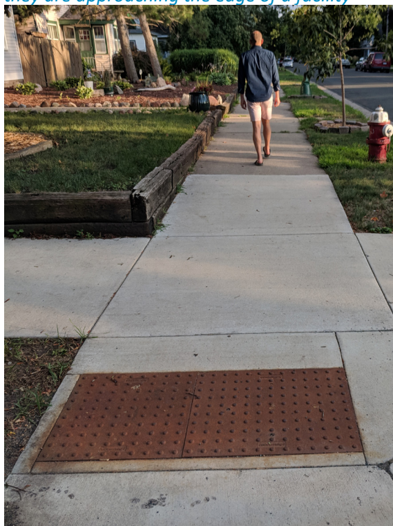
Figure 3-6: Detectable warnings alert users that they are approaching the edge of a facility
