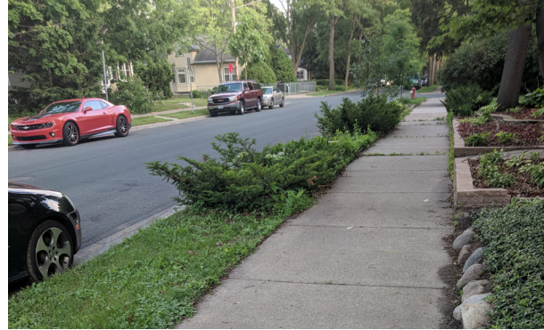
Figure 3-15: Typical residential sidewalk section with grass boulevard
