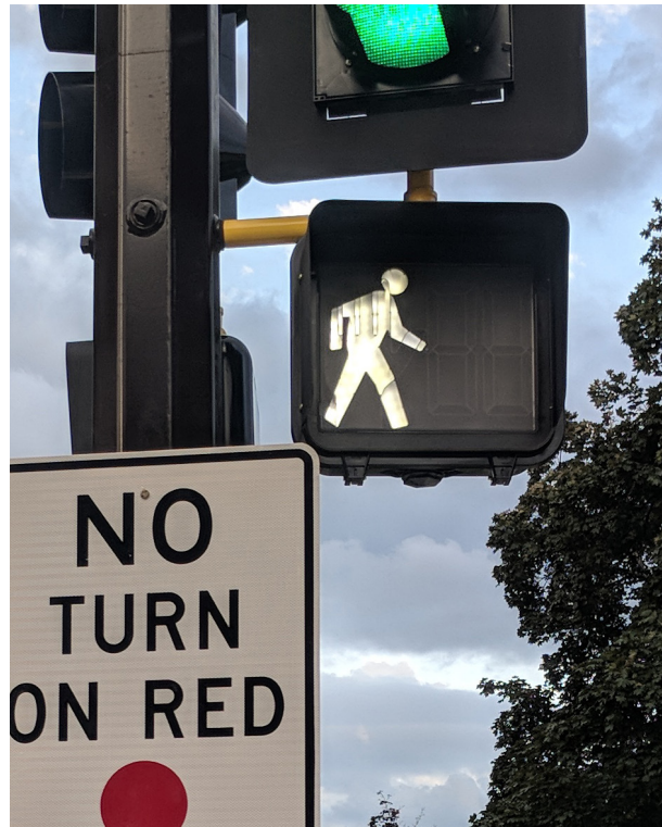
Figure 4-9: Pedestrian signal head
