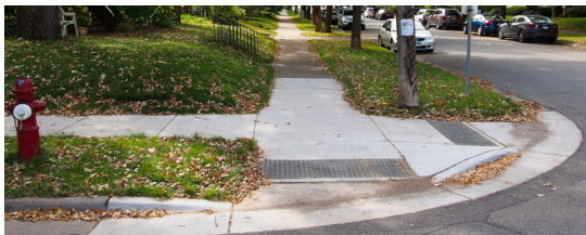
Figure 3-2: Combined Directional Pedestrian Curb Ramps provide two separate ramps at each corner
