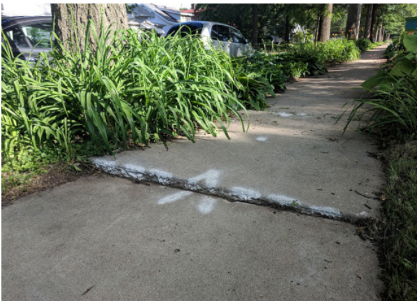
Figure 4-11: Uneven sidewalk
