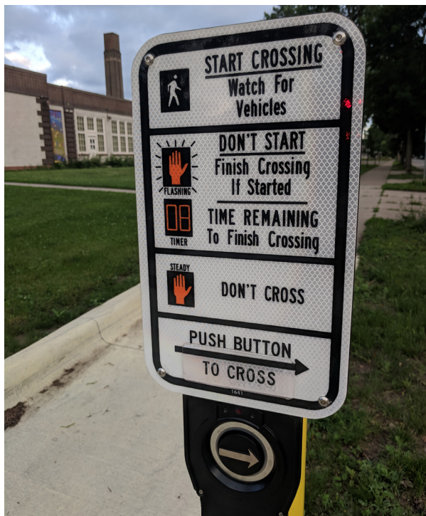
Figure 4-8: Accessible Pedestrian Signal (APS) push button
