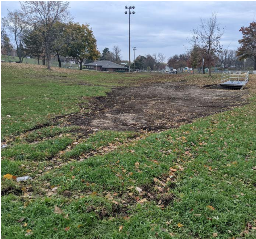
Sibley dry pond - Bare soil due to construction
