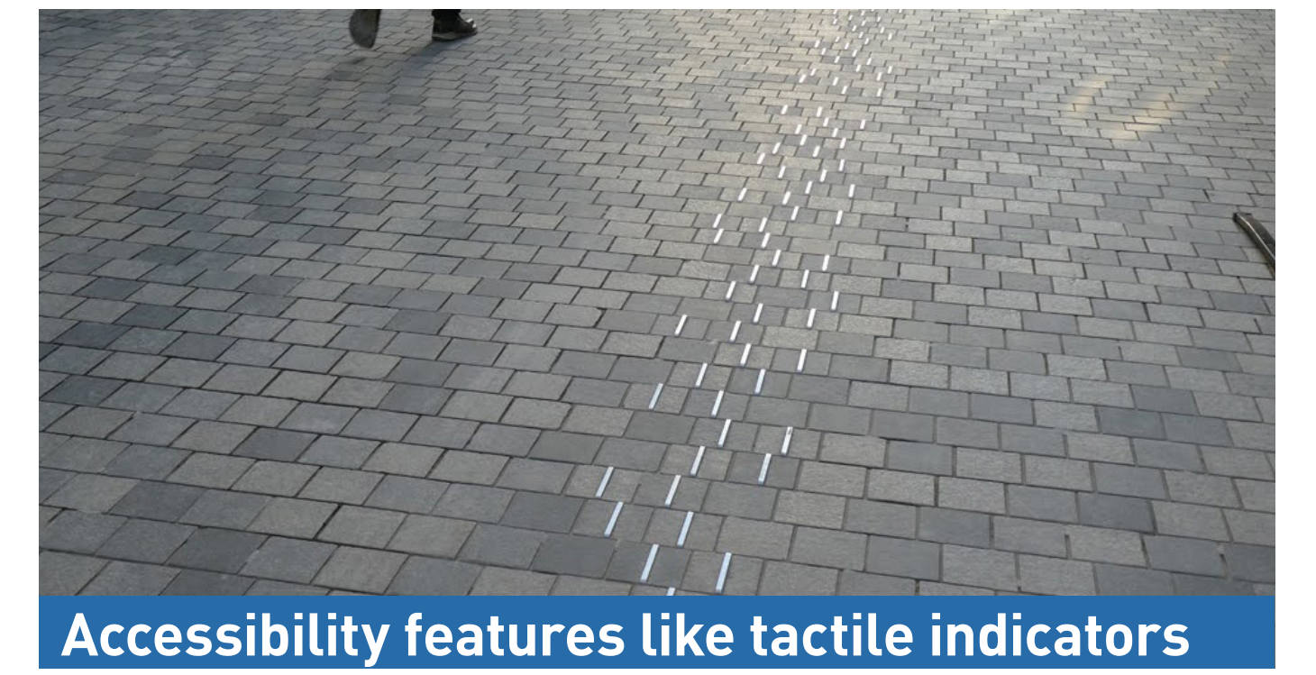
Accessibility features like tactile indicators
