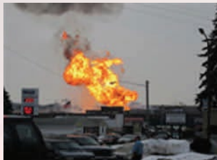
Natural Gas Leaks
