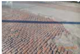
Logan Park pavers were installed on their "stretcher" side
