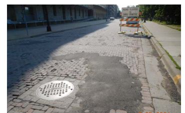
Manual repair of concrete pavers are labor intensive and still failed 8 years later at Main St SE - which had only a 15-year life.
