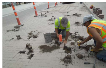
Manual repair of concrete pavers are labor intensive and still failed 8 years later at Main St SE - which had only a 15-year life.
