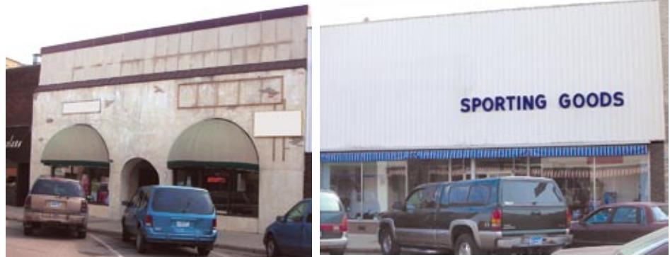
BEFORE The aluminum siding on the sporting goods store conceals the unique architectural details and cornice of the building. This is discouraged.
