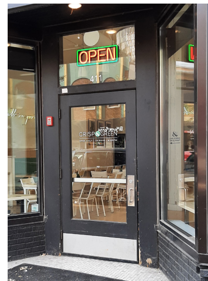
Here is a replacement door at 411 14th Ave SE. Metal doors with glazing are appropriate in this historic district.
