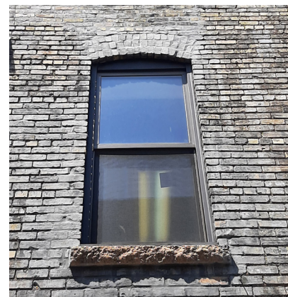
This window has a brick arch above and a stone sill below. Lintels, pediments, moldings, and hoods are typically found around the tops of windows.
