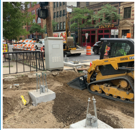
Grading for sidewalk work at the 1st Ave. N intersection.
