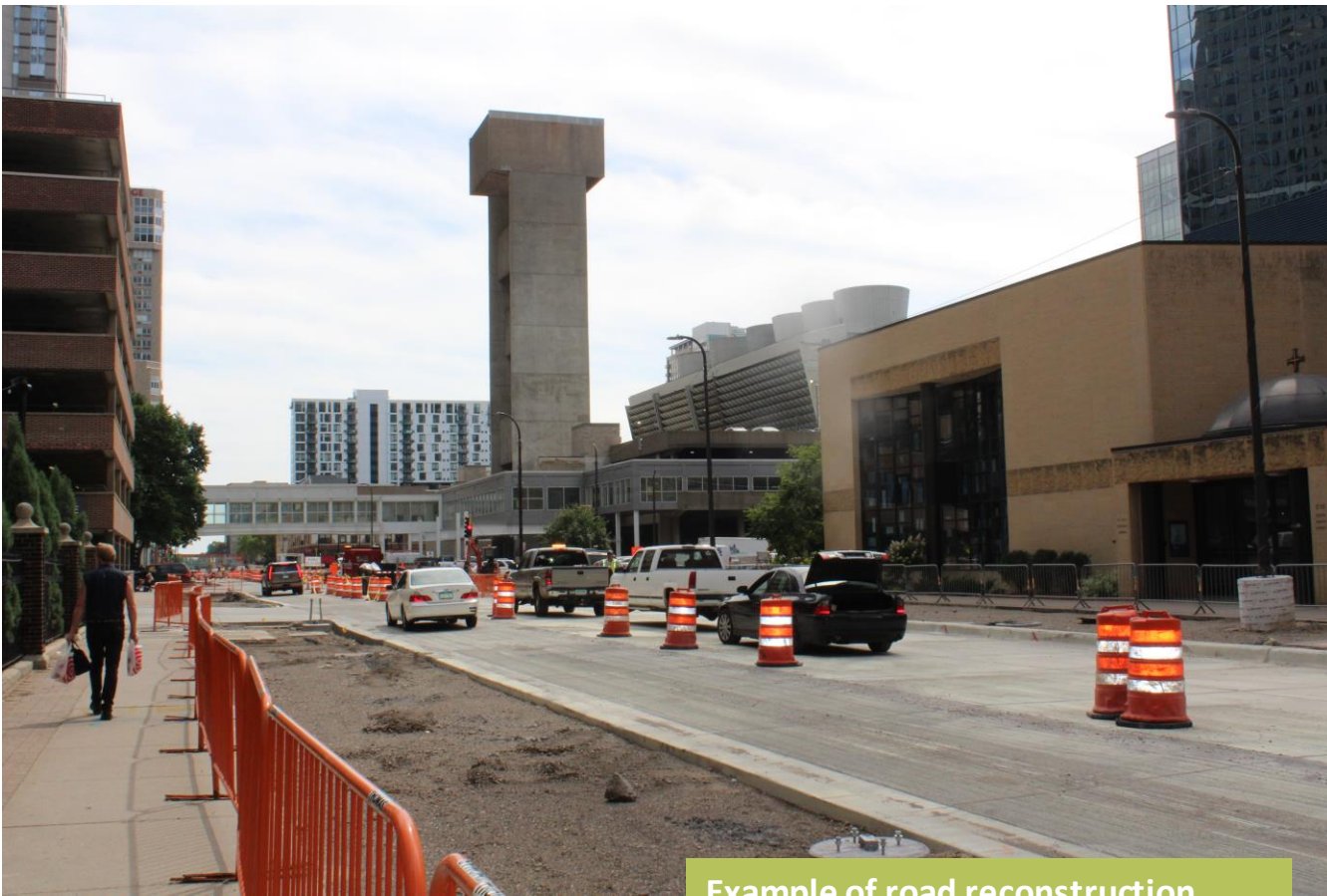
Example of road reconstruction
