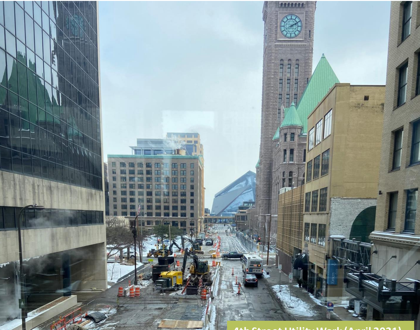
4th Street Utility Work (April 2021)
