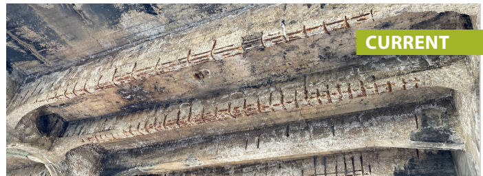
Deteriorating concrete and reinforcing on bridge underside
