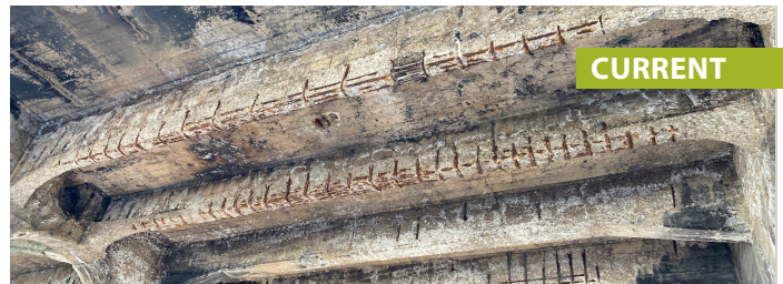
Deteriorating concrete and reinforcing on bridge underside
