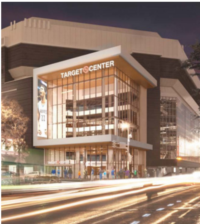
Target Center Renovation
