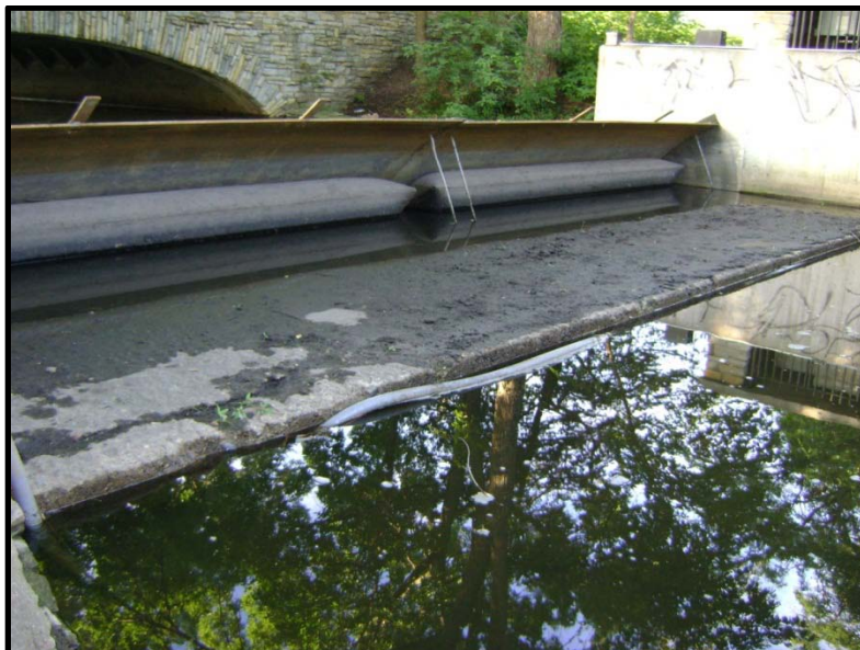
View of Inflated Weir from the "Creek" Side of the Structure
