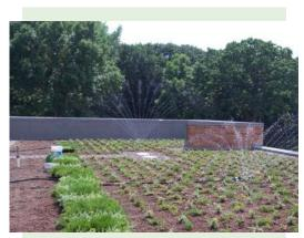
The facility's living green roof drastically reduces water runoff and provides superior insulation for the building.
